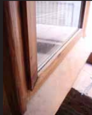
6-06_23_double glassing bathroom
