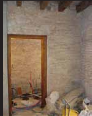
2-06_15_bathroom from bedroom
